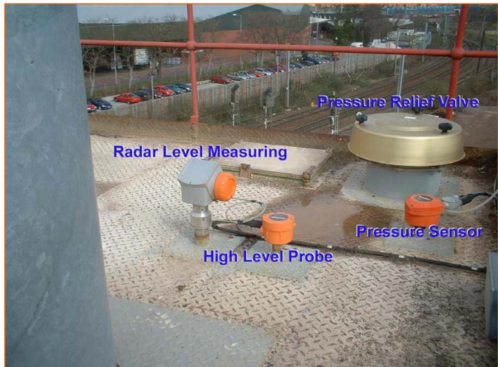
will fit in the silo. Where only a high level probe is fitted, the SiloSafe GLT will automatically check its operational integrity. If a high level condition is reached during filling, warning is given via the siren and
