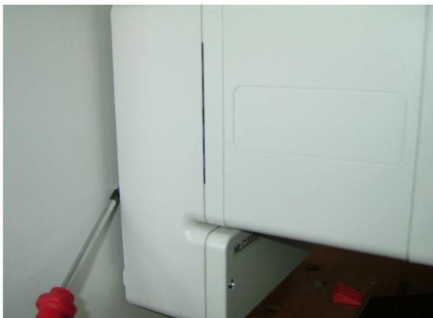
Secure controller to brackets by tightening screws.
