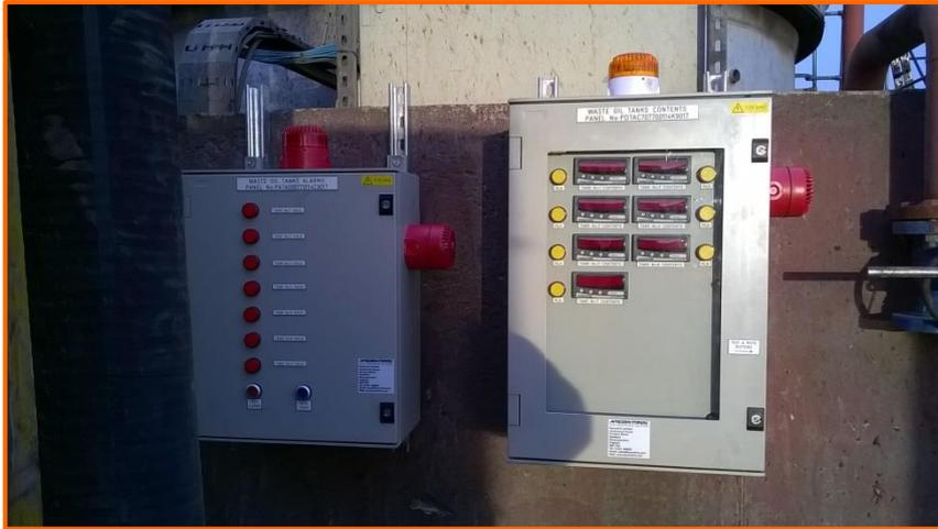
connected to a designated Hycontrol alarm panel, activating visual and audible alarm should levels in any tank rise above a pre-determined level. This duality provides a 'belt and braces' approach should anything affect the reading from the TDR system. The
