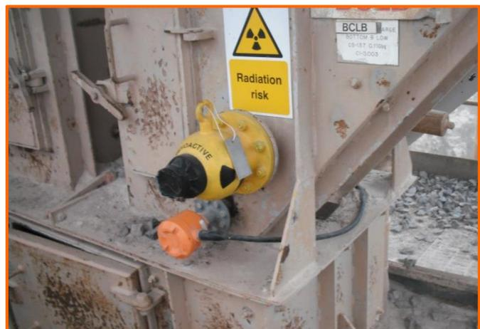
Hycontrol's new generation of microwave switches is proving to be an extremely reliable, robust and cost effective alternative, offering operators a 100% safe solution for blocked chute detection. This range of microwave level switches provides a simple non-contact, non-intrusive option suitable for
