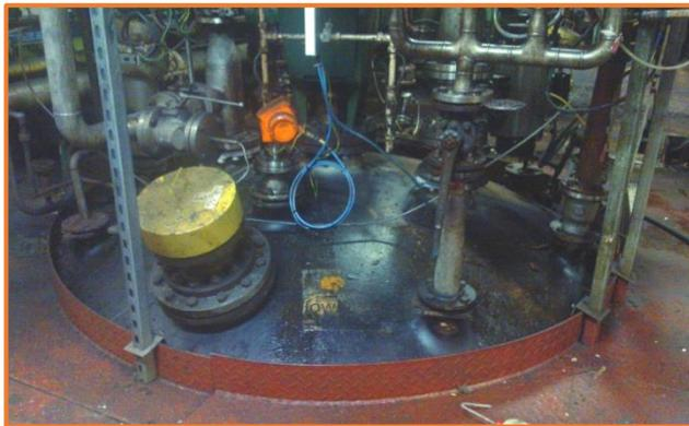
Based on extensive experience in such applications, Hycontrol engineers were confident their ATEX compliant VG7 radar level measuring system with drop antenna and DiFoam non-aqueous foam probe and control system would meet the dual challenge of accurate tank contents measurement and improved foam control with reduced de-foamer consumption. As
