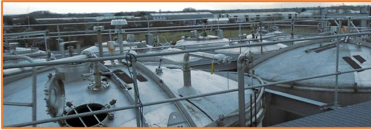
ATEX-certified level measuring equipment installed by **Hycontrol** is providing important contents monitoring data and overfill prevention at **Centec International's** chemical storage farm in Cheshire.
