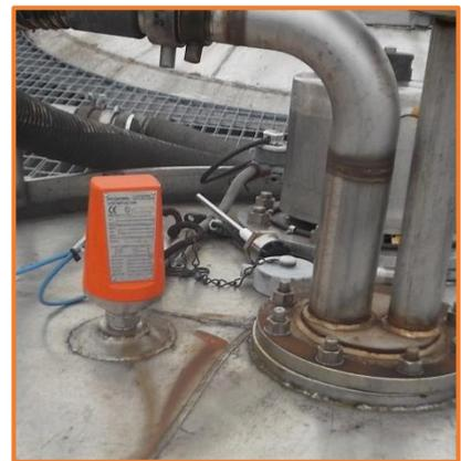
Initially Hycontrol's ATEX-trained engineers fitted TDR sensors via flanges at the top of four of the tanks, with the stainless steel conducting probes extending down to the bottom of the vessels. These were connected to a bespoke 16 point instrument and alarm panel, located 35 metres away in the weighbridge office within the safe zone.
