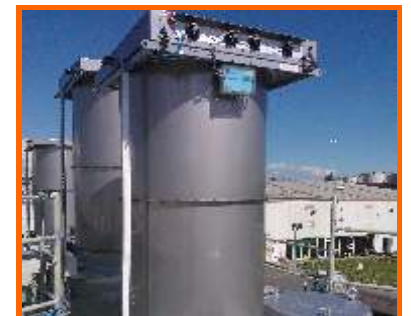
New reverse-jet filters fitted
