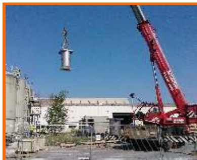
Complete project installation
