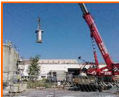
Complete project installation
