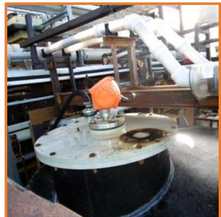
Hycontrol range of radar technology products and provide exceptional levels of accuracy over a maximum range of 80 metres.
