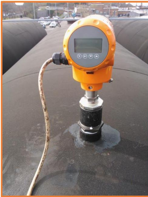
TDR devices, which have a dead zone of just 150mm. This provides an ingenious solution to overcome the restricted headspace between the bottom and top tanks. Whilst a fixed sensor antenna or probe is designed to fit the overall depth of the tank in one piece, the coaxial rod sections can be assembled incrementally as the probe is inserted into the tank via the process connection. The sensor software converts measured depth to volume based on the tank profiles.
